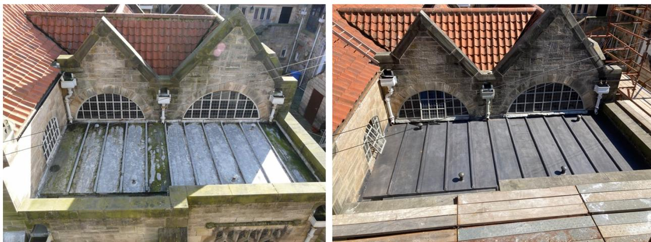
What are you looking at? This is the roof over the Sacrament Chapel and the west end of the south aisle. As a rule of thumb with lead roofs, dark grey colours are good, white is not good, and green is worse. New lead is treated to change it from silver to dark grey to prevent the process that leads to a build-up of reactants that slowly 'rot' the lead to a white, powdery compound that is little use for keeping buildings dry.
